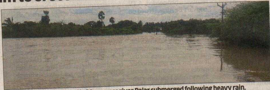
The ground-level bridge across river Palar submerged following heavy rain.
