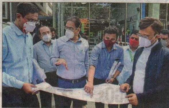
BBMP Administrator Gaurav Gupta inspecting the progress of pipeline work in Koramangala Valley on Wednesday.
