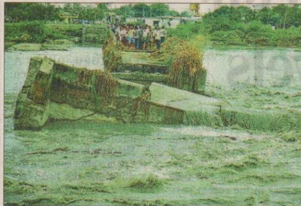
A retaining wall (bandara) across Hirehalla collapsed due to heavy rain as a result of which water gushed into nearby villages.
