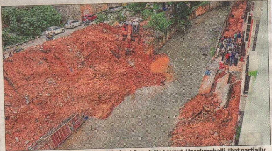
The retaining wall of a stormwater drain at Gurudatta Layout, Hosakerehalli, that partially collapsed following the rains. The BBMP is building a temporary wall there. DH PHOTO/PUSHKAR V
