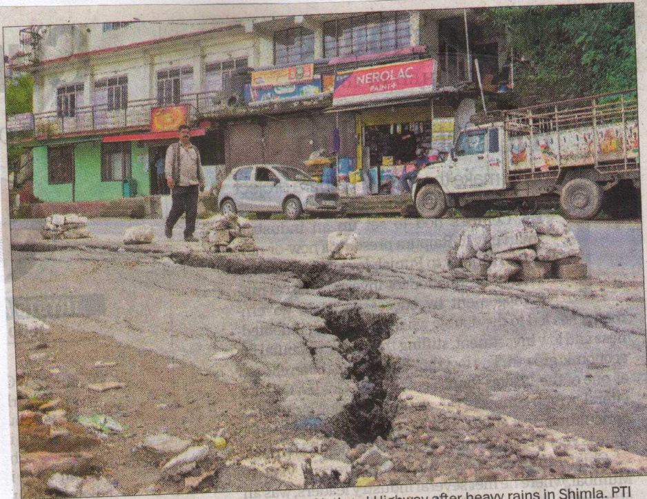
Cracks appear on the Shimla-Chandigarh National Highway after heavy rains in Shimla. PTI
