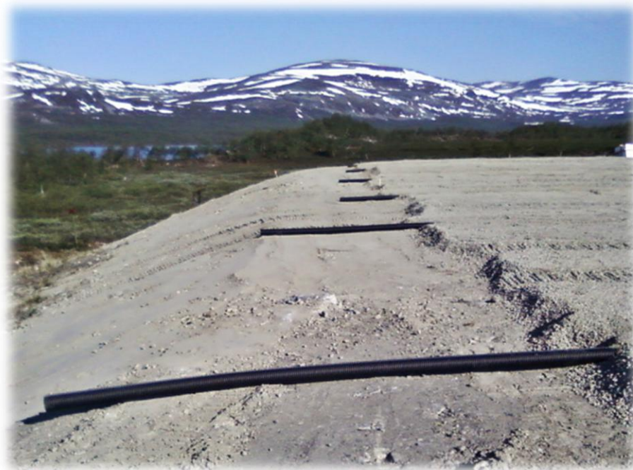
Figure 3-7: Provision of drain pipe
