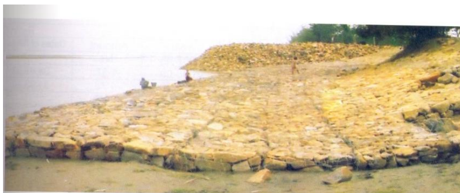
Figure 4-8: A typical bank pitching in wire crates
