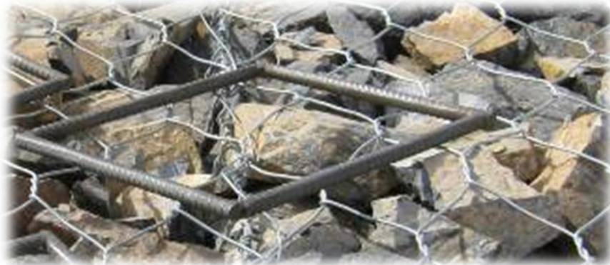
Figure 8-8: Boulders filled in gabions
