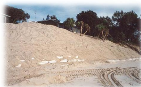
Figure 4-13: Bank after implementation of geo-bags
