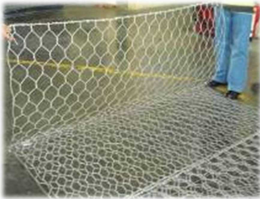
Figure 8-4: Straightening out of DT mesh panels of folded gabion unit
