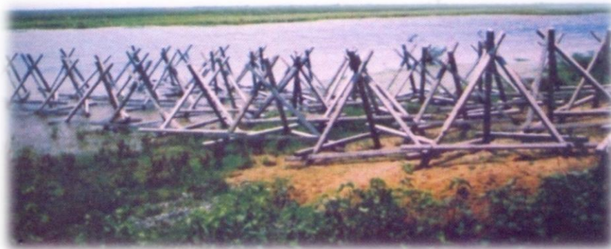
Figure 6-4: RCC porcupine spur
