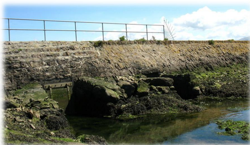
Figure 7-4: A gated sluice
