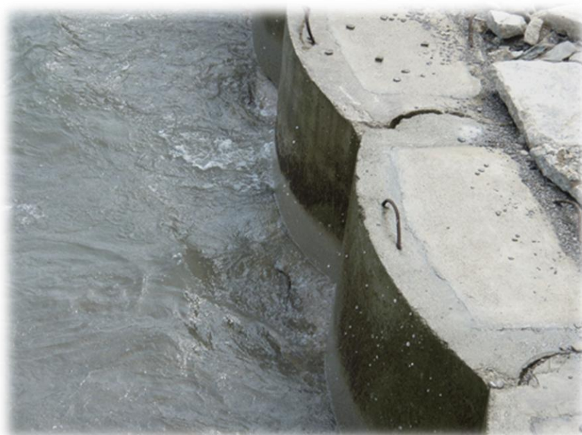
Figure 4-11: Use of cement blocks in bank protection
