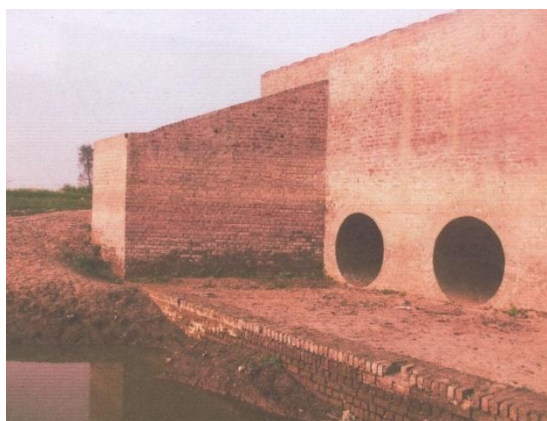
Figure 7-1: A cross drainage work
