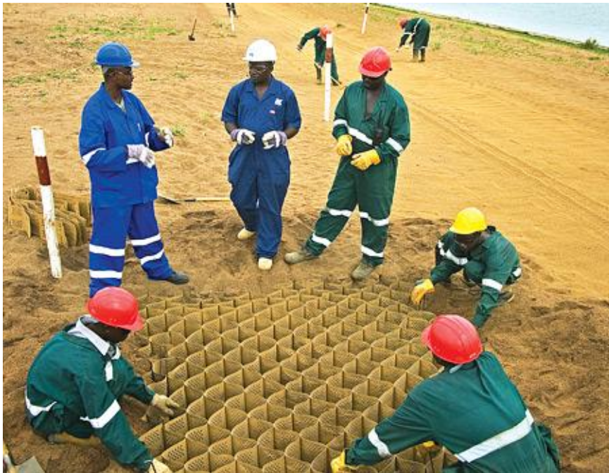
Figure 4-7: A typical geo-cell being prepared at site
