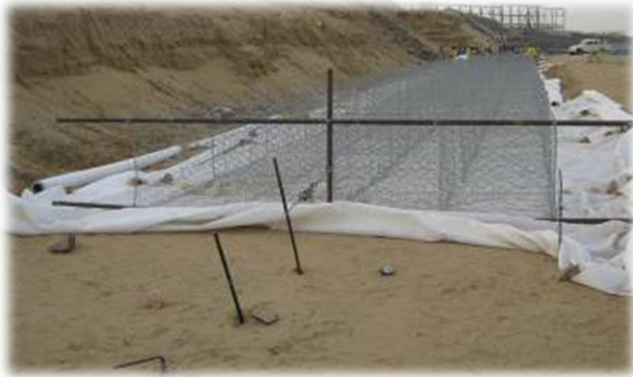
Figure 8-7: Stretching the gabions
