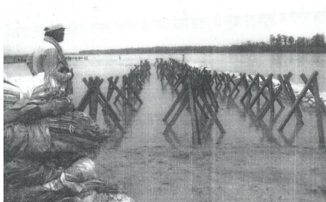
Figure 5-8: A typical RCC porcupine spur
