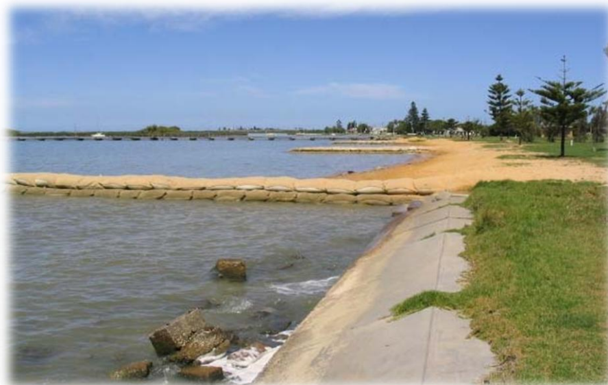
Figure 5-7: Spur along with bank protection using geo-textile
