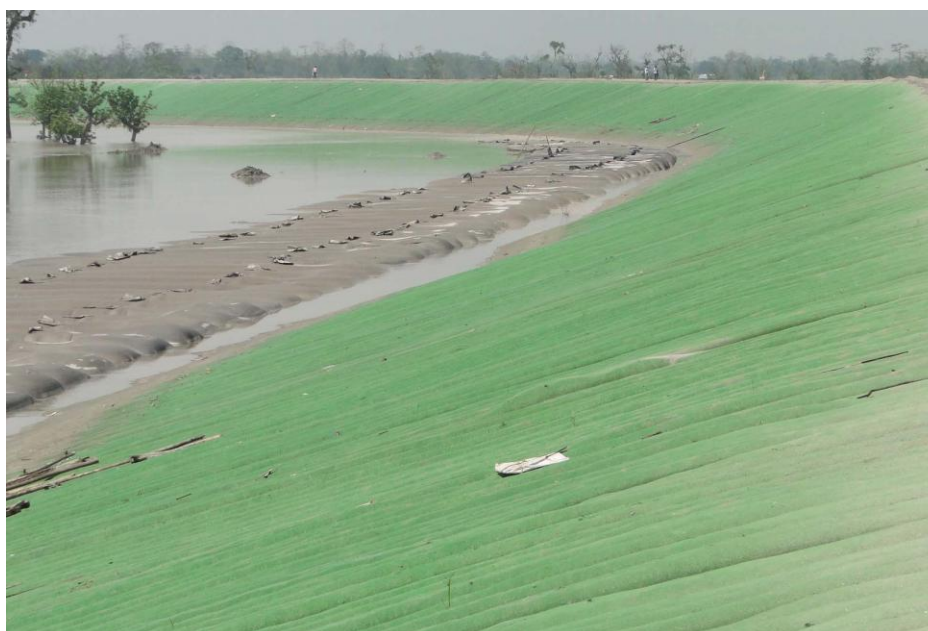
Figure 3-1: Typical high embankment with slope protection using geo-mattress
