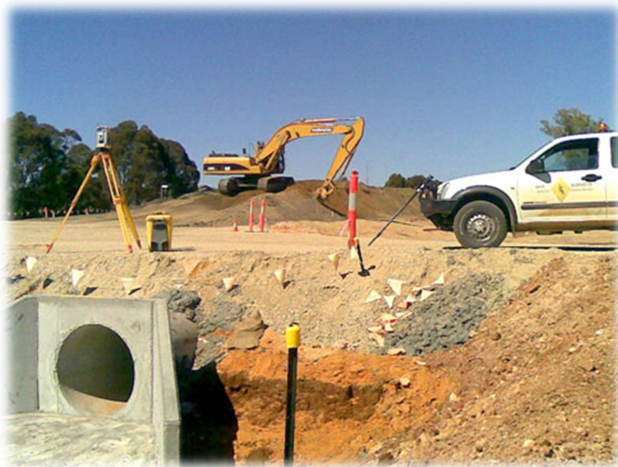
Figure 7-2: cross drain under the embankment
