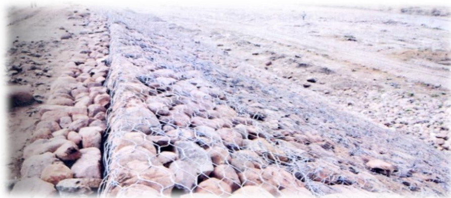
Figure 4-9: A typical bank pitching in crates
