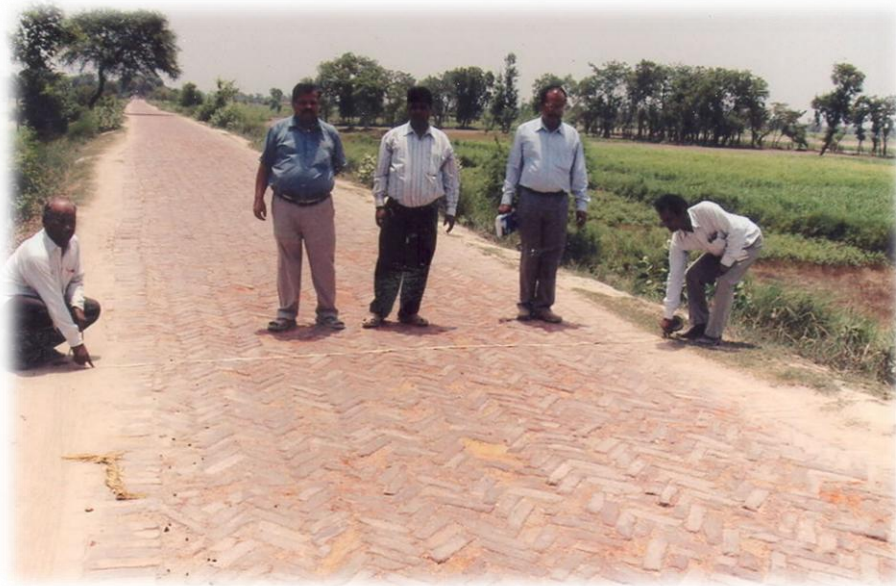
Figure 3-4: An embankment crest with brick soling
