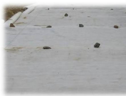
Figure 8-3: Geo-textile laid out on rolled surface
