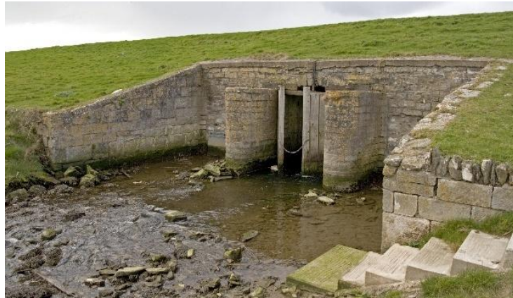
Figure 7-6: A typical gated sluice drain
