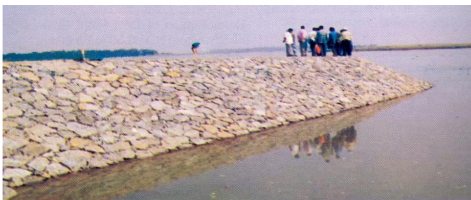
Figure 5-1: Spur built with boulders
