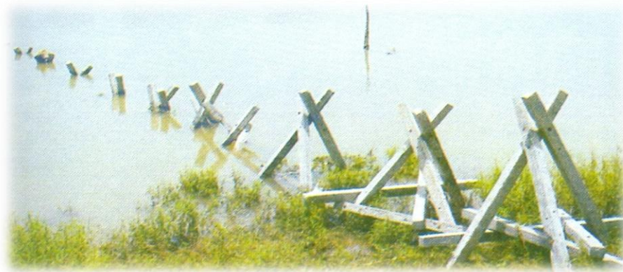
Figure 6-2: Typical RCC porcupine screen
