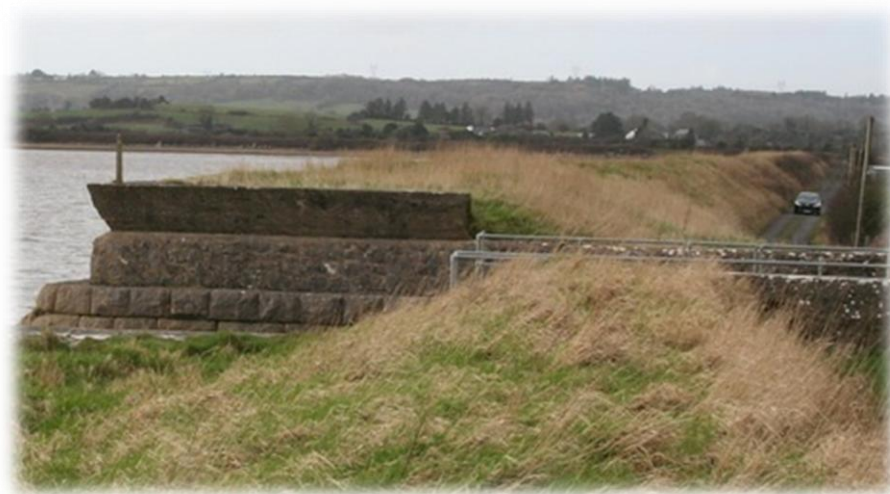
Figure 7-3: Embankment with sluice
