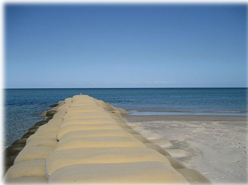
Figure 5-6: Spur using geo-bags
