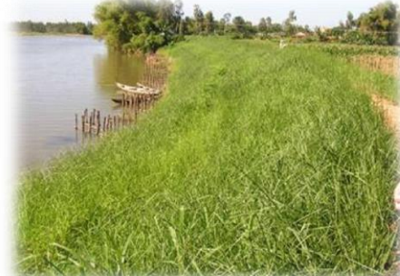
Figure 4-4: Bank after the vetiver implementation
