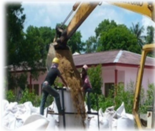
Figure 8-11: Filling of geo-bags
