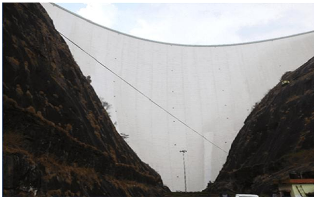
Upstream Reflective Coating at Idukki Dam
