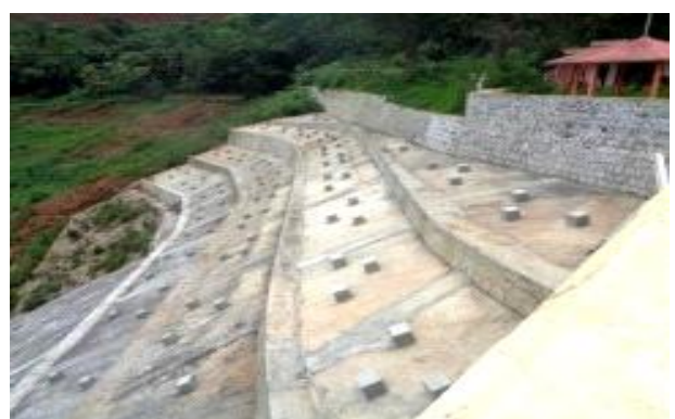
Earth Slip Soil Erosion Protection Works
