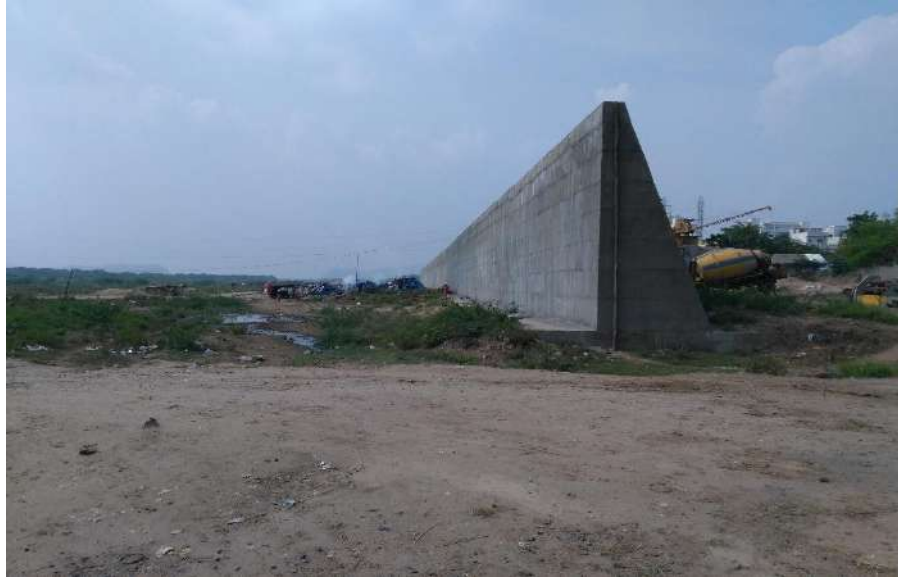
Fig. 99: Cantilever retaining walls constructed on the right bank downstream of Prakasam barrage; upstream view
