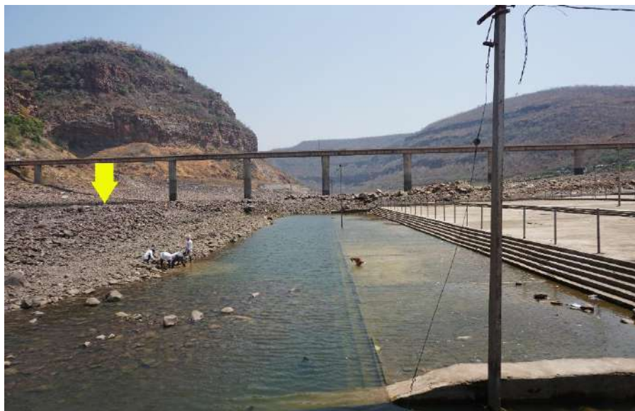
Fig. 94: Aggradation of channel bed in KR_17 (downstream of Srisailem dam) after 2009 flood
