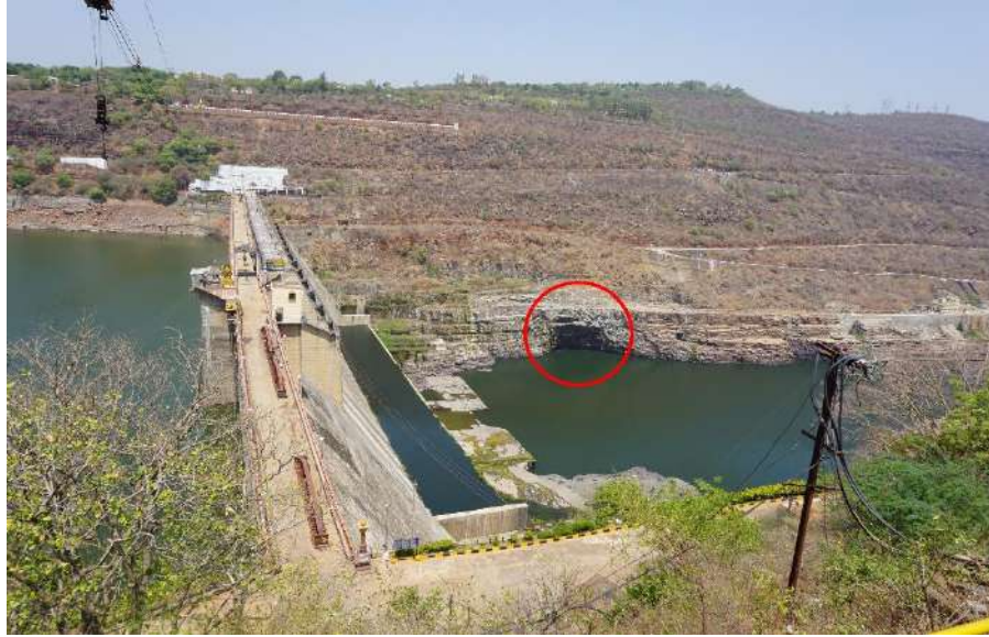
Fig. 79: Scouring occurred on the left bank channel wall in KR_17 during the 2009 flood; view towards NNE
