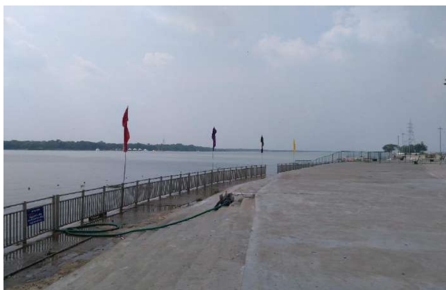
Fig. 98: Berms constructed on the right bank of KR_22, upstream of Prakasam barrage
