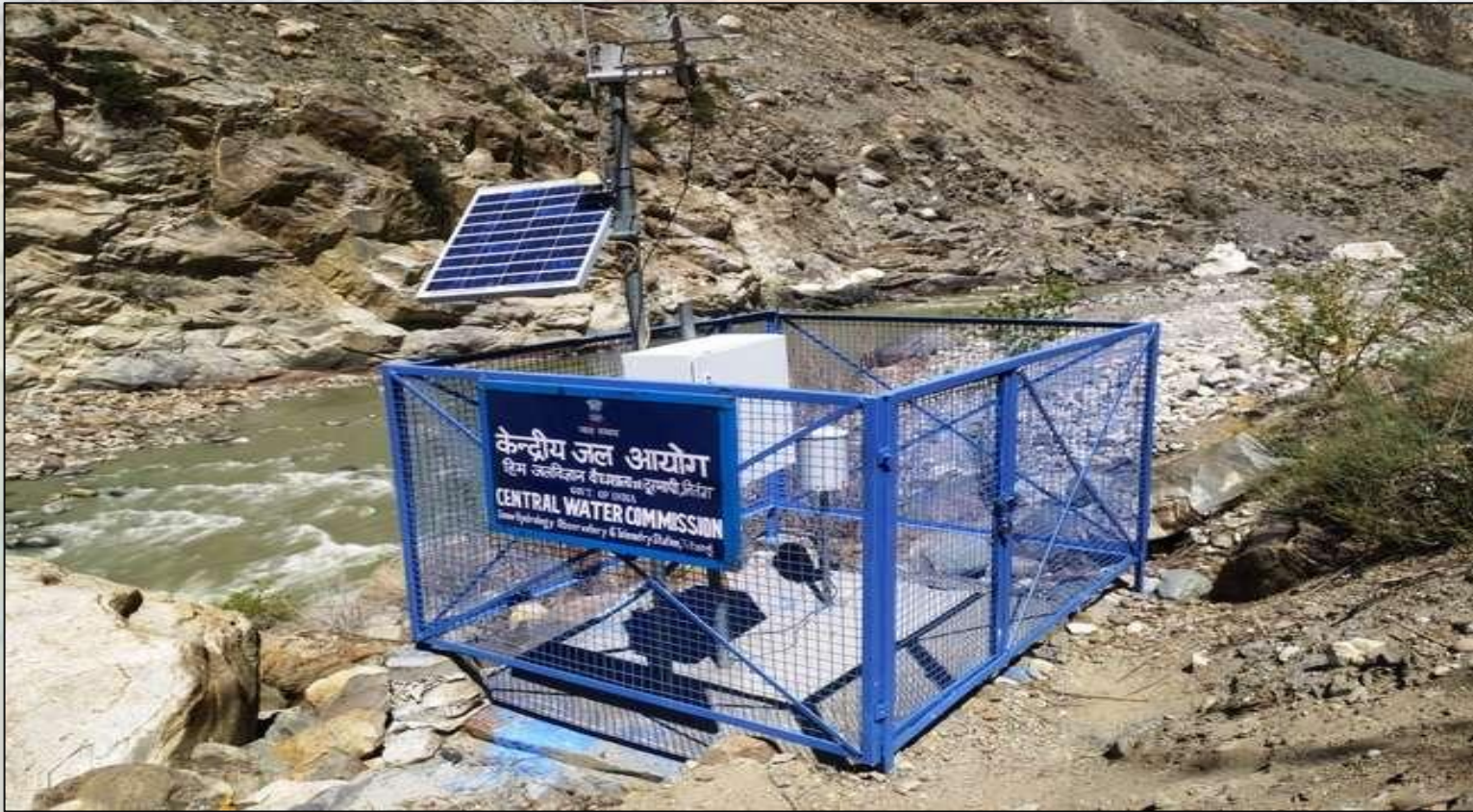
TITANG B-TYPE TELEMETRY STATION, SHD, CWC, SHIMLA ON RIVER SATLUI
