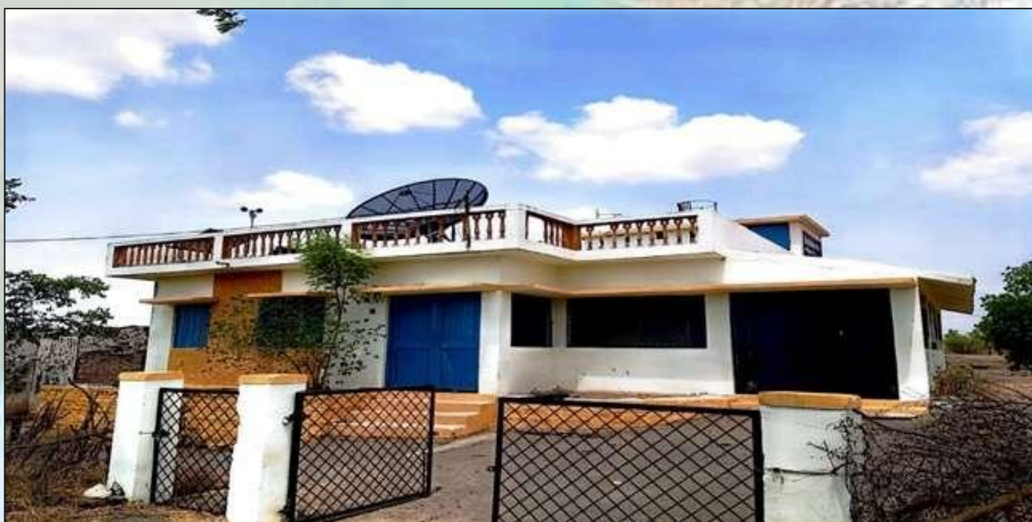
SITE OFFICE- DHULSAR ON URI RIVER UNDER, INDORE
