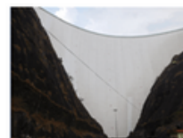
Upstream Reflective coating at Idduki dam
