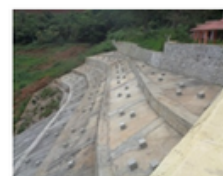
Earth slip soil erosion protection works
