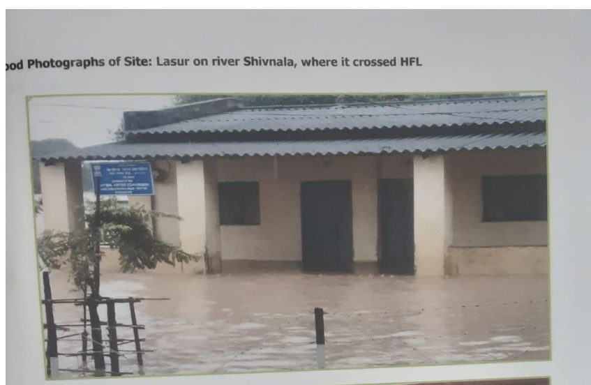
Lasur on River Shivnala, Andhra Pradesh Floods 2021
