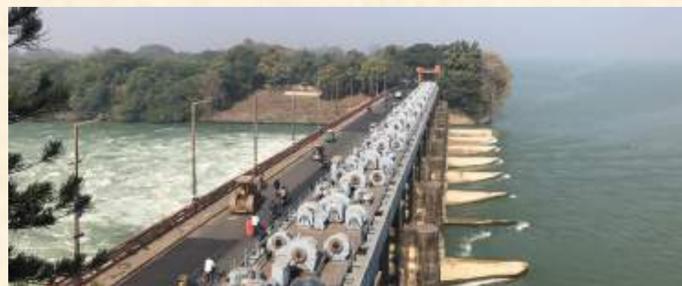
Farraka Barrage (1975): Head regulator comprises of 11 numbers of gates for diversion of approx. 40,000 cusec of discharge into 38.3 km long feeder canal.
