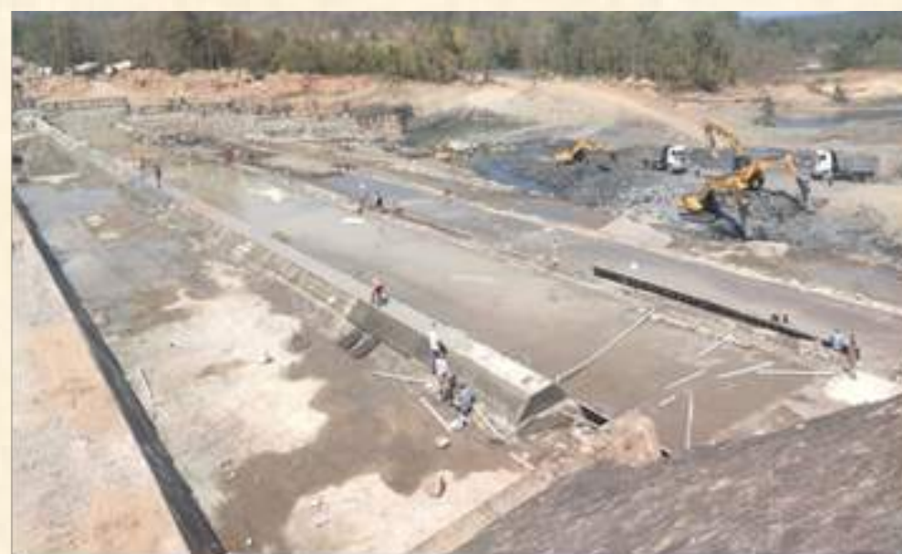
Sikasar Dam Chhatisgarh: CWC provided design and drawing for rehabilitation of eroded spillway.
