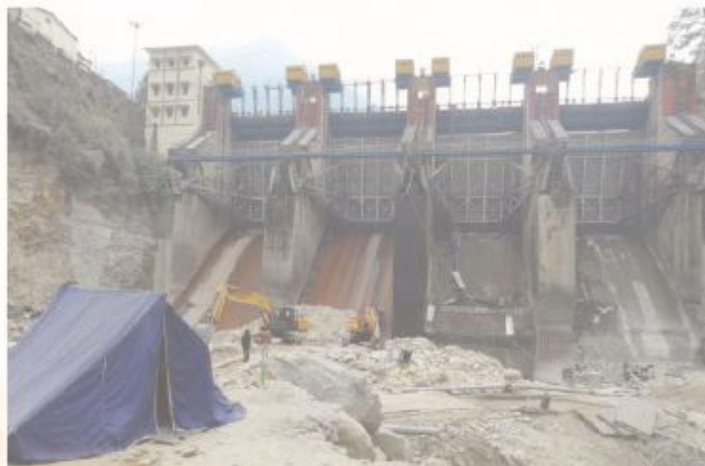
Repair of spillway glacis and energy dissipator with M90 concrete (Maneri Dam, UJVNL)
