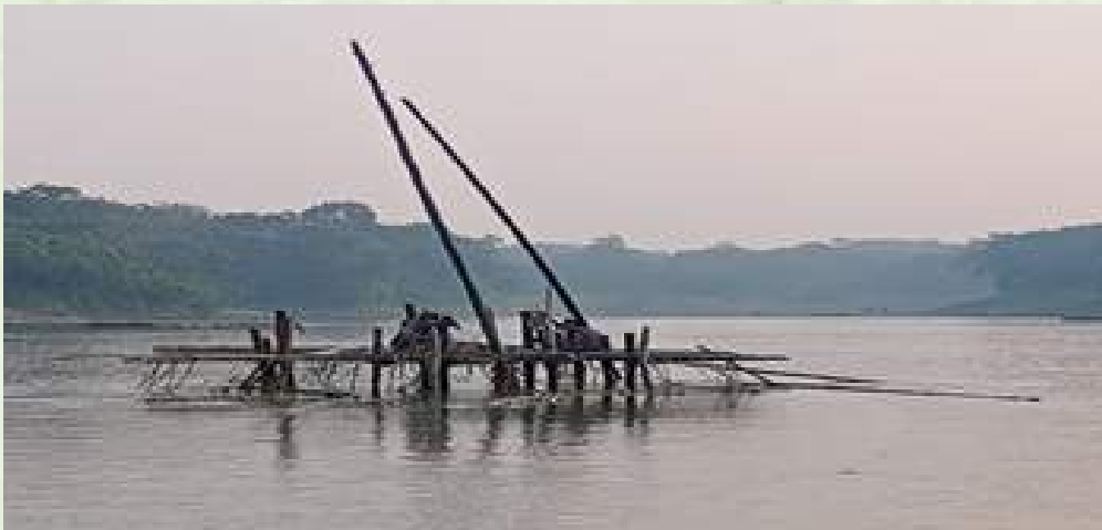
Diamond Core Drilling at Katakhal Irrigation Project as a part of subsurface investigation.
