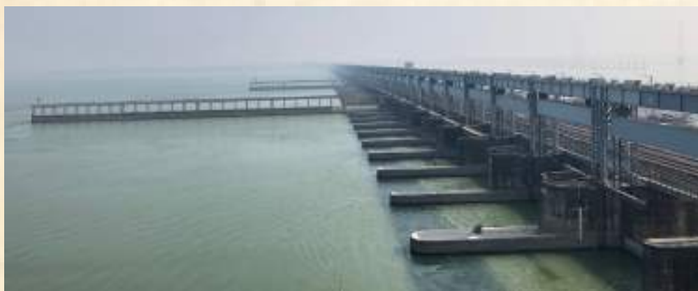
Farakka Barrage Project, W.B. (1975): is an important diversion project crucial for implementing international water treaty between India and Bangladesh. The Barrage is 2305 m long and comprises of 112 numbers of gates. It provides water to Calcutta port and is the only rail link between North East and rest of India.
