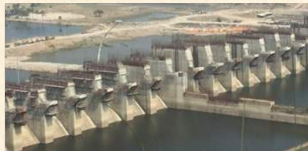
Polavaram Irrigation Project, Andhra Pradesh: (Under construction) CWC approves the design for Civil and Hydro-Mechanical works.
