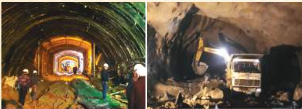
Fig. 6 Central gullet tunnel excavation in diversion tunnel of Arun III HEP (900MW), Nepal; Mucking after blasting in tunnel
