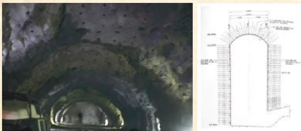
Fig. 9 Excavated crown of powerhouse cavern of Arun III HEP (900MW), Nepal in January 2020 (left). Spot bolts installed immediately after excavation are visible; Rock support system of the powerhouse cavern as envisaged (right)
