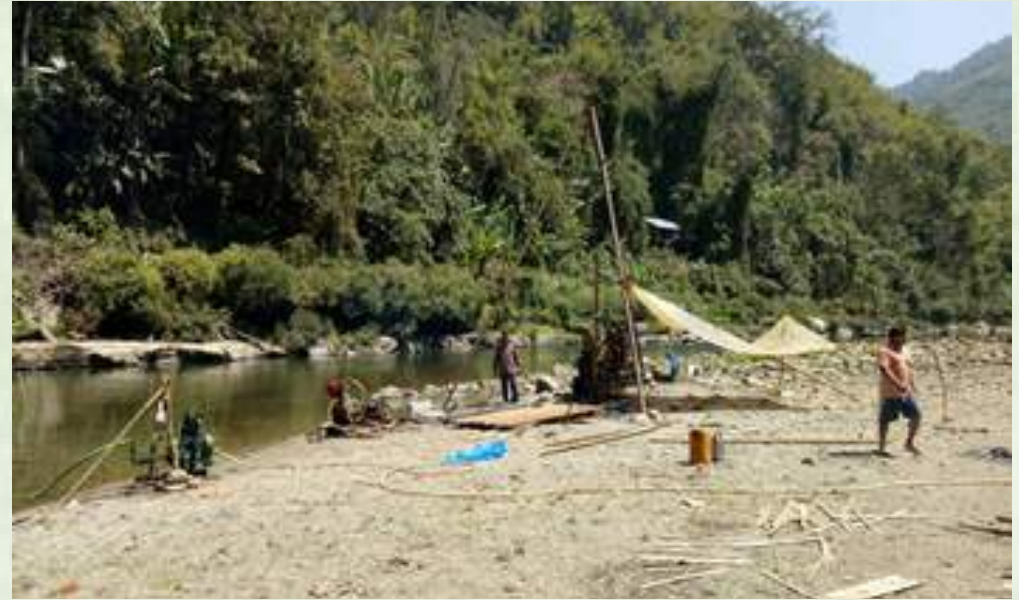
Drilling work at mid of the dam axis at Tlawng HEP, Mizoram to obtain the depth at which rock strata is available
