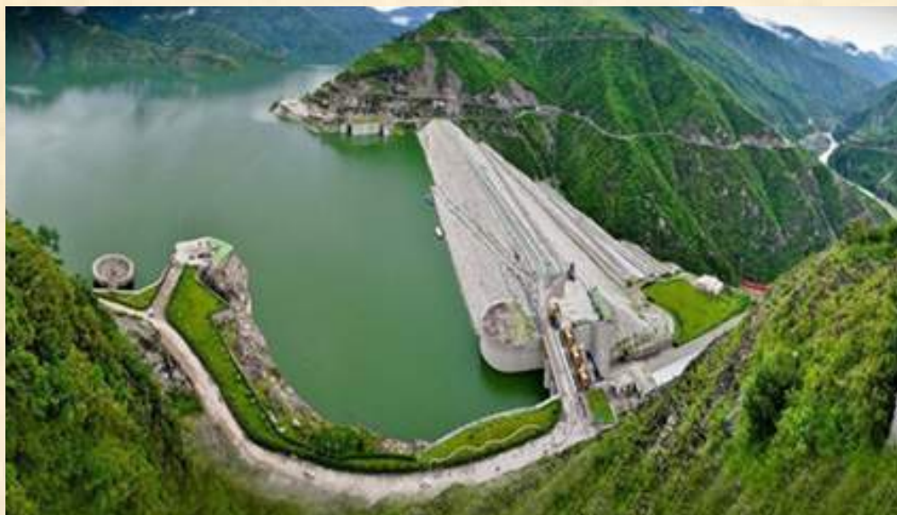
Tehri Dam Project, Uttarakhand (2006): CWC has been associated with the planning and design of various components of the Project. The design engineering for dam, Chute Spillways, Shaft Spillways, Intermediate Level Outlets, etc. was done by CWC.
