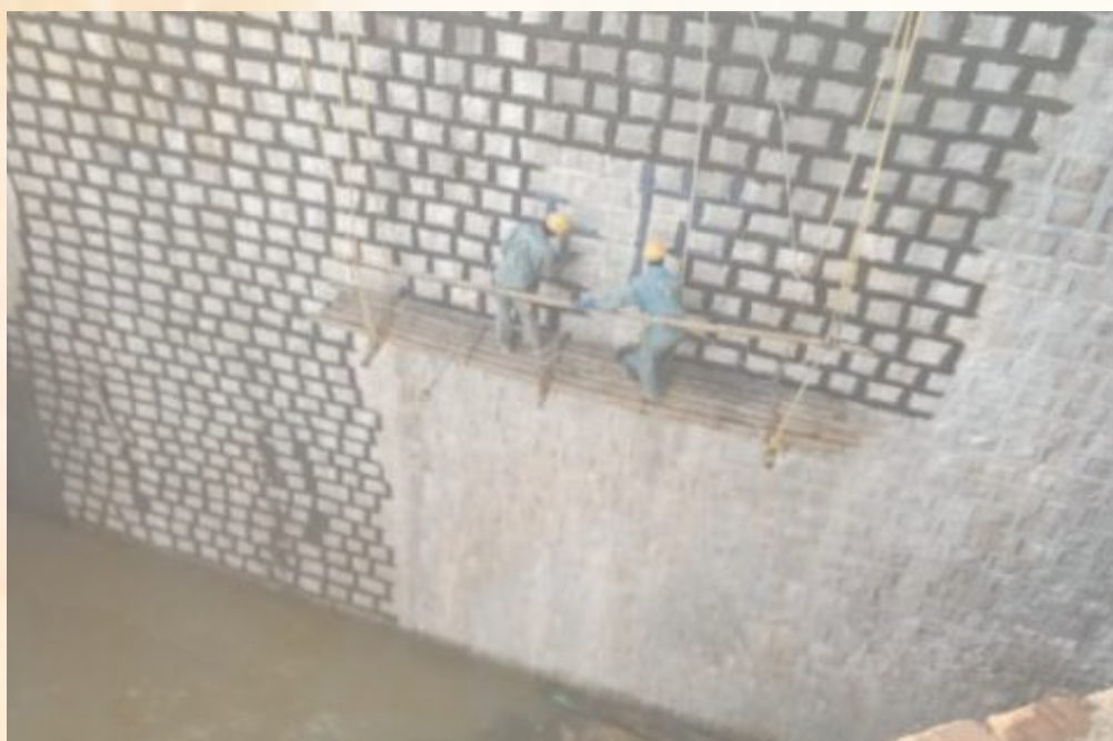
Racking & pointing of upstream face with UV resistant, high strength crystalline technology including underwater (Malaprabha dam, KaWRD)
