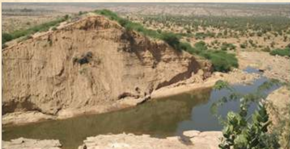
Garada Dam Rajasthan: CWC provided technical assistance for rehabilitation of its breached portion.
