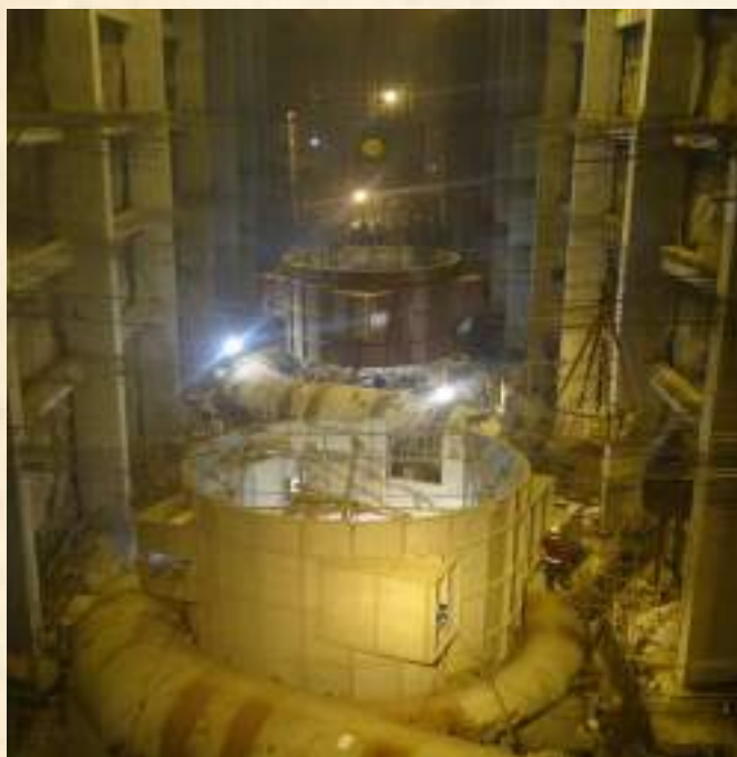
Underground Power House-Machine Hall Punatsangchu-I H.E. Project (1200 MW), Bhutan: CWC is the design consultant to this ongoing project.
