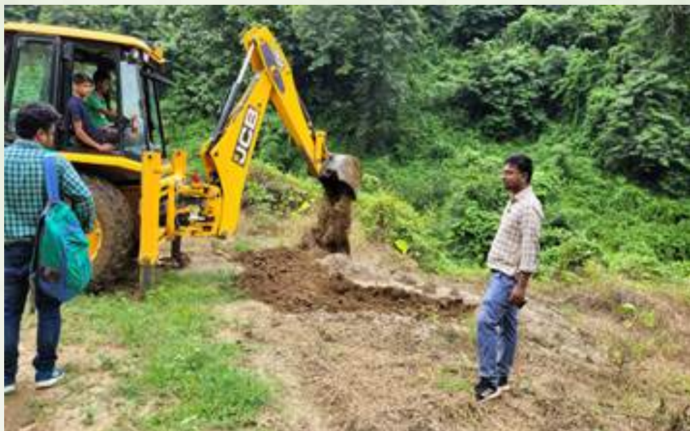
Collection of soil sample from Borrow Area of Haora Dam Project in West Tripura with CSMRS officials.
