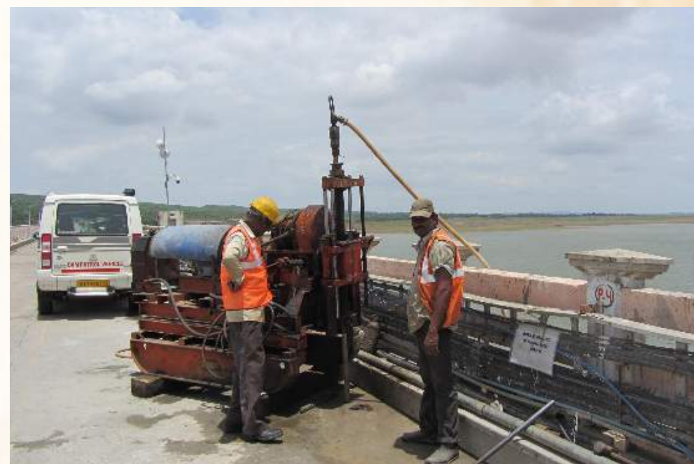
Dam body grouting with mix of cement, micro-silica (Almatti Dam, KaWRD)
